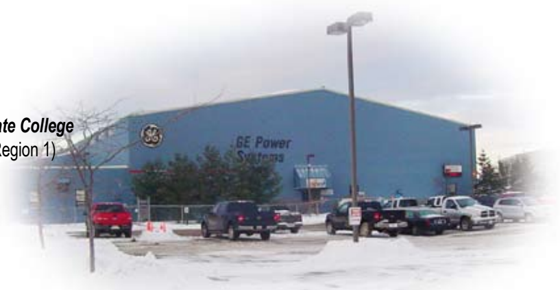
GE Energy 534 Griffin Road • Bangor, Maine
